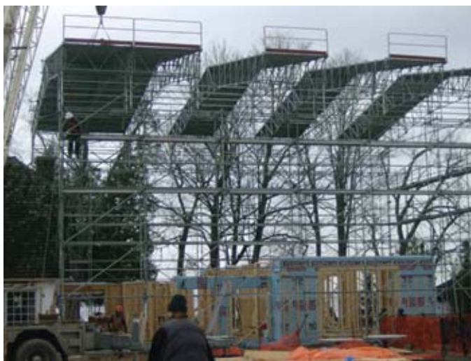
Roof being hoist onto system scaffold.
